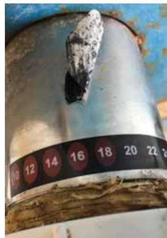
Figure 1a: Temperature strips placed on the water outlet
